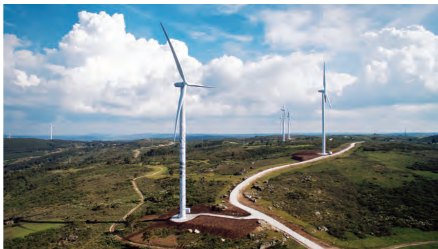
With the permission of Finerge
