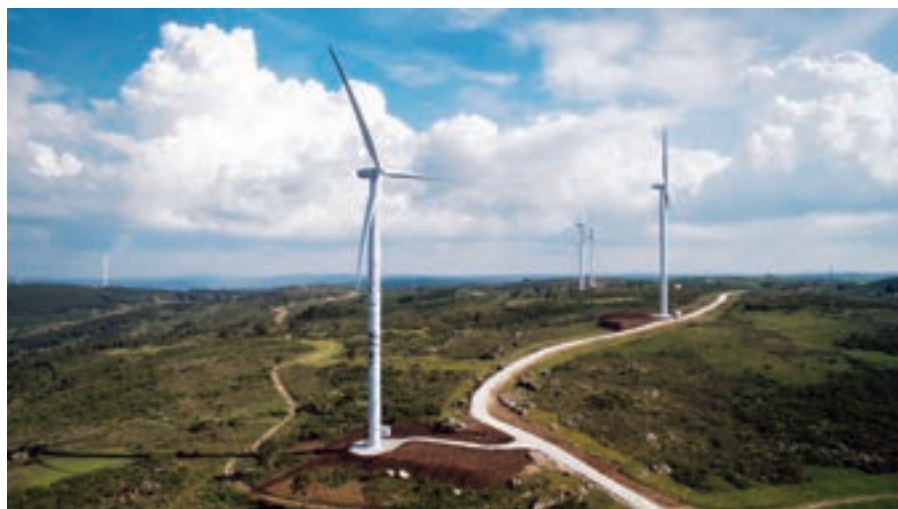
With the permission of Finerge
